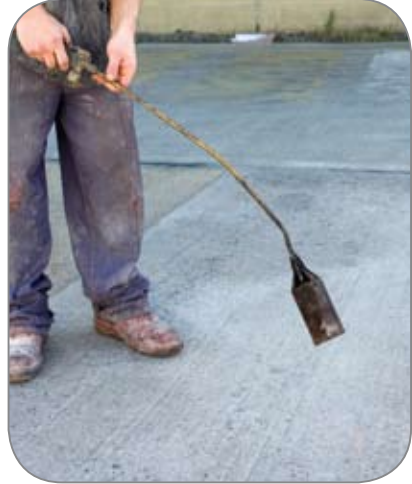
Drying with hot air lance
