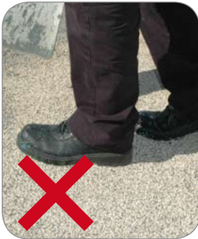
Do not walk on aggregate or resin
