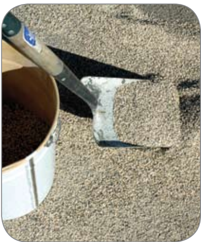
Collect any excess aggregate
