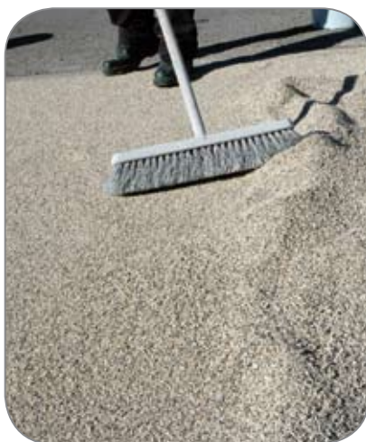
Excess aggregate brushed off
