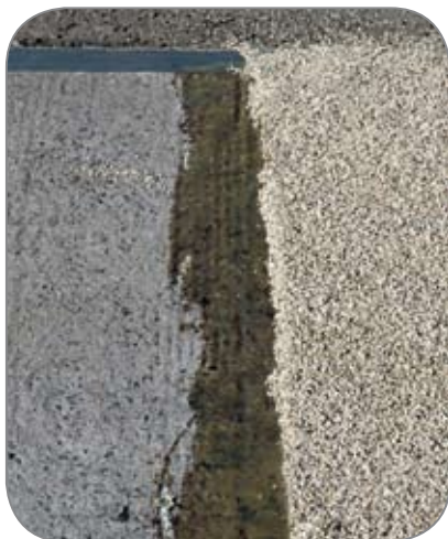
Wet edge left for adjoining area
