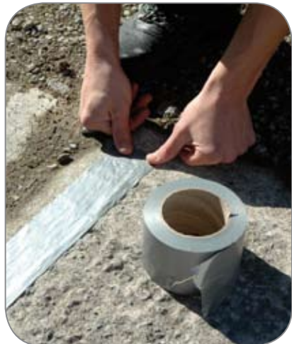
Masking-off with peelable tape
