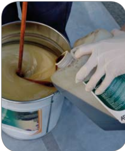
Add activator slowly whilst mixing
