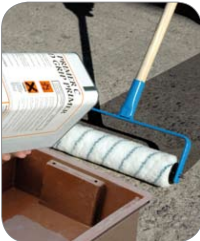
Use Primer C on absorbent surfaces
