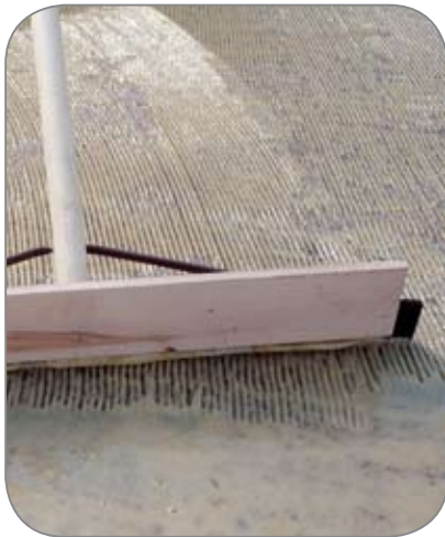
Spreading and regulating
