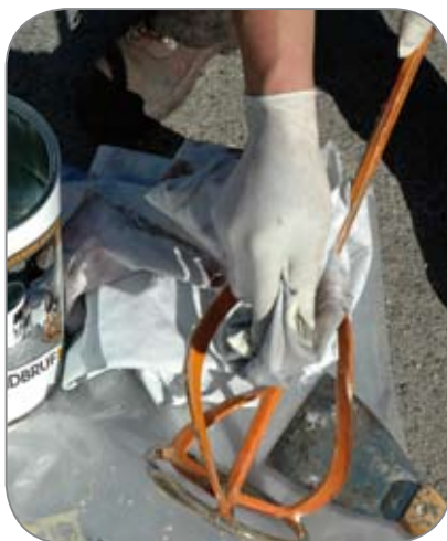
Equipment cleaned with solvent
