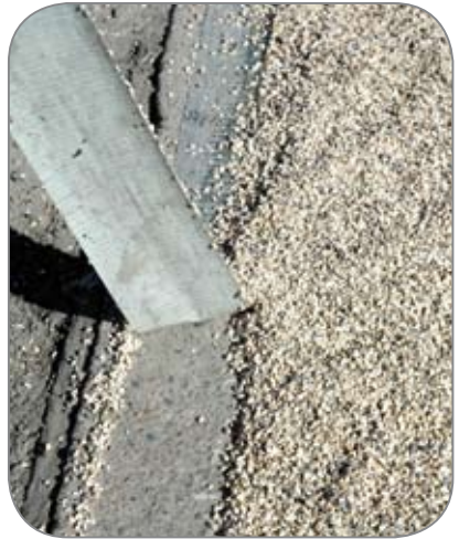
Masking tape being removed
