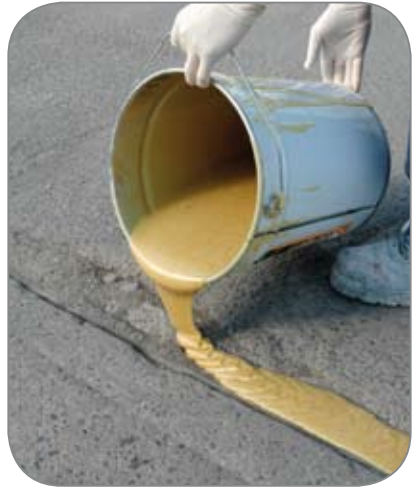
Laying material in flowing lines
