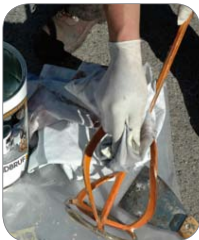
Equipment cleaned with solvent
