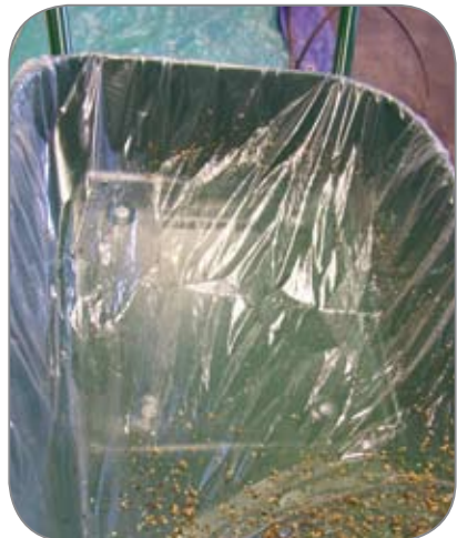
Pour mix into polythene lined wheelbarrow
