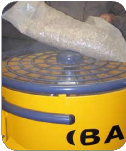
Charge the mixer with aggregate
