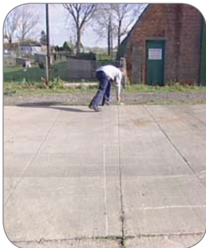
Concrete slab joints
